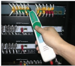
Copper cabling detecting
